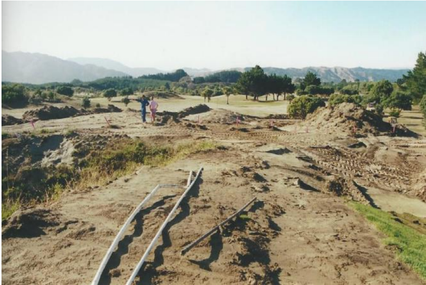
New 16 th tee under construction
